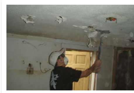
Beginning the demo work
