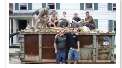
A very full dumpster
